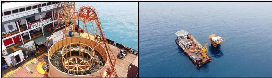
Replacement 15KV 500MCM Subsea Cable – Pertamina Hulu Energi OSES.
